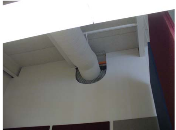
Open beam and duct penetrations
