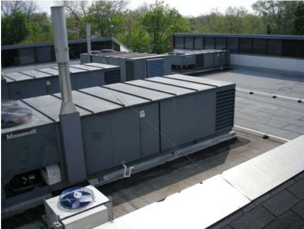
Gas Fired Multizone Rooftop Unit
