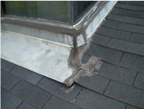
Damaged flashing and sealants
