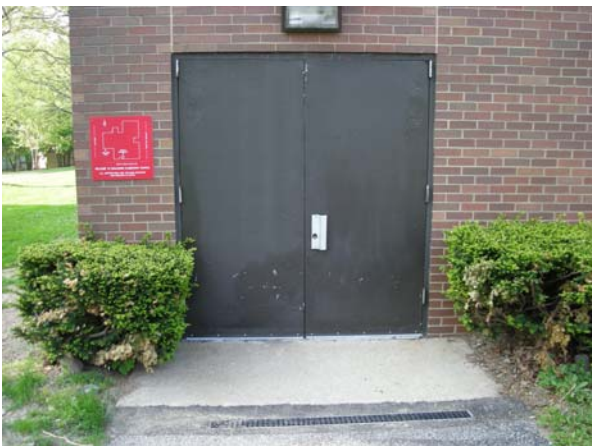
Typical exterior door condition
