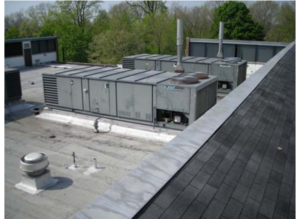
Gas Fired Multizone Rooftop Unit
