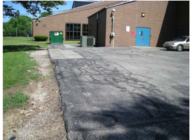
Repeatedly damaged and repaired asphalt
