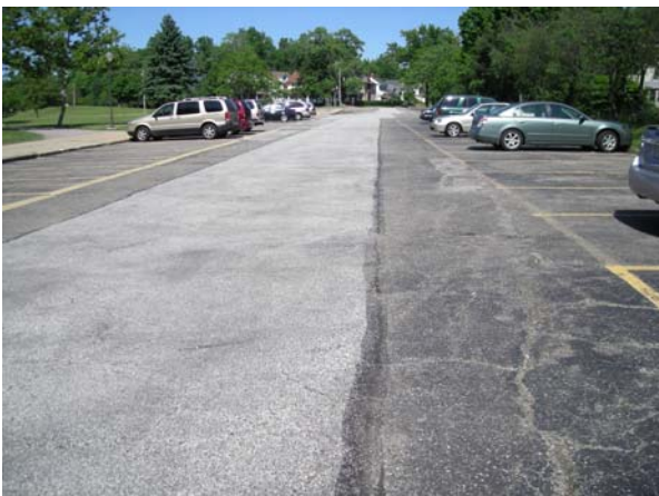
Damaged asphalt in parking lot
