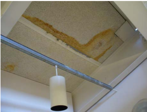
Water damage to ceiling
