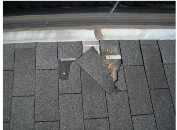
Damaged asphalt shingles
