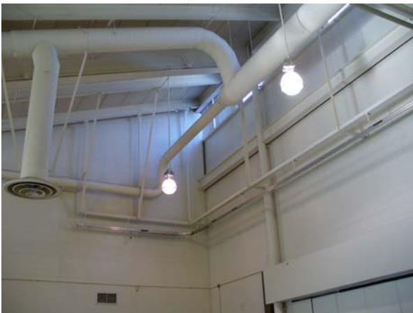
Typical Exposed Ductwork
