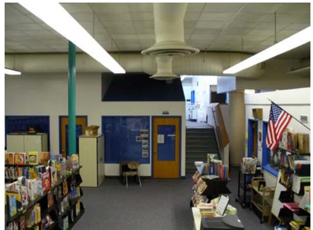
Typical Exposed Ductwork
