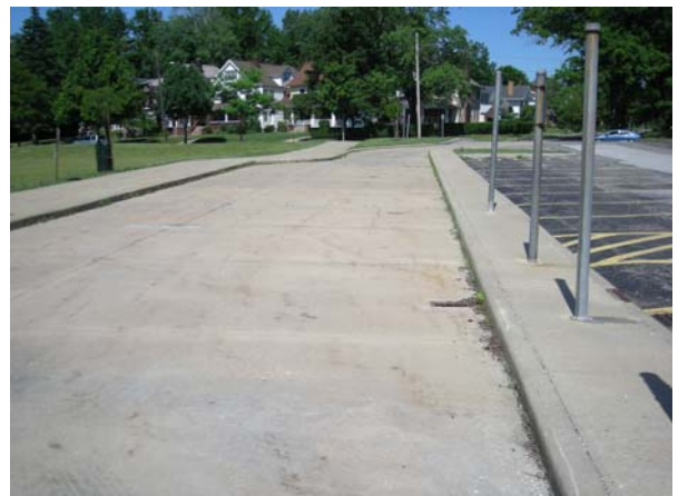
Damaged concrete at bus dropoff
