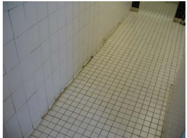
Damaged tile walls and base
