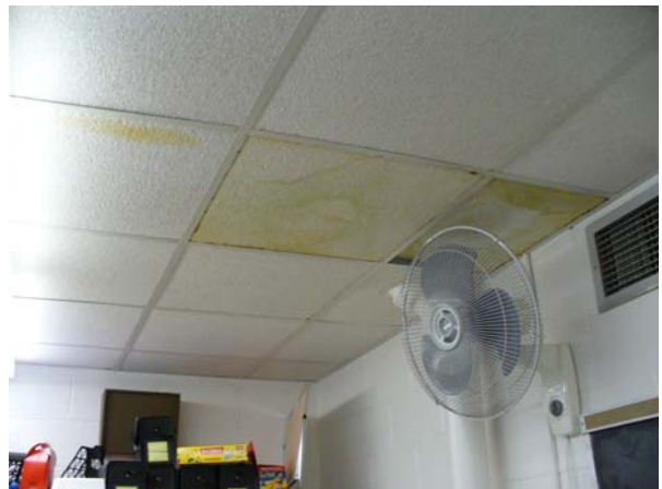
Water damage to tile ceiling
