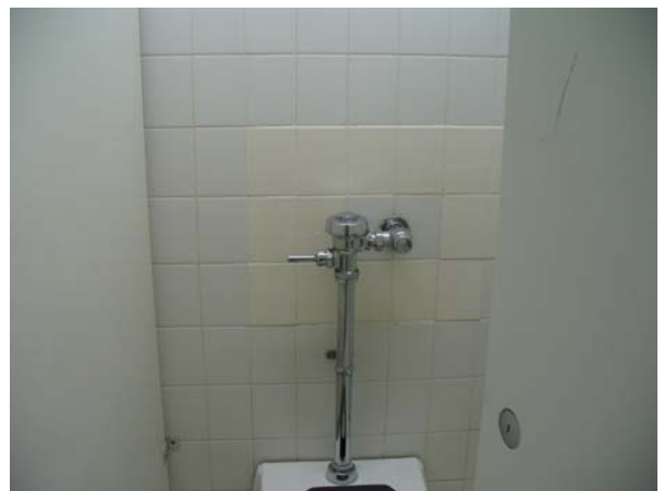
Tile wall repair
