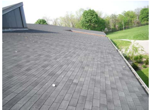
Roof deck deflection
